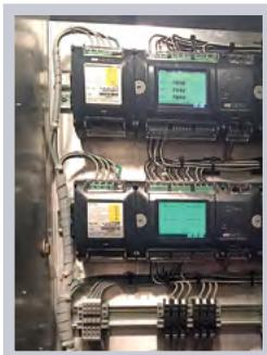
The BFM-II is designed to upgrade legacy substations featuring electro-mechanical (EM) relays, to provide real-time information and control over these highly reliable, yet limited, devices.
