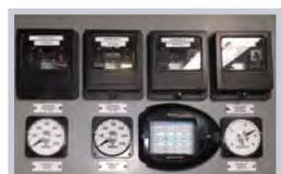
One BFM-II monitors up to 18 three-phase circuits located up to 200m/650ft away from the device. The BFM II utilizes unique split-core High Accuracy Current Sensors (HACS) that simply clamp around the secondary wiring of the existing 5A secondary of the protection CTs. This eliminates the need to interfere with the protection circuit, eliminating the need for a full shutdown or interruption of the substation.
